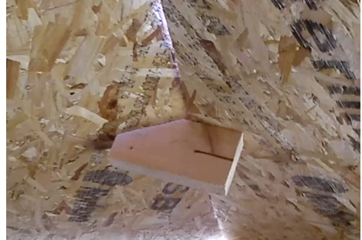
150° block joining roof pieces
